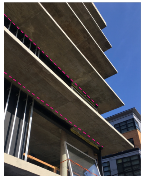
Non-Repeating Thermal Bridges Included separately from the U-Value
