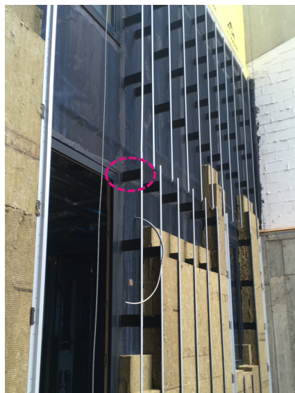
Repeating Thermal Bridges Included as part of the U-Value
