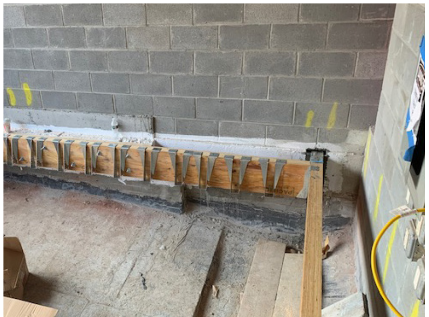
Install the structural ledger and the floor joists. Note that in the case shown here, the ledger is supported by two beams which do pocket into the masonry and which are carefully sealed at all edges. See the next section for beam-pocket details.
