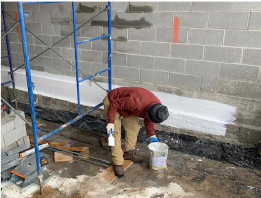
Apply the liquid air-seal material to the ledger zone and ensure that it extends far enough on all sides that it can be continued across the wall in later steps.
